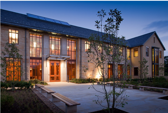
The exterior of the library.
